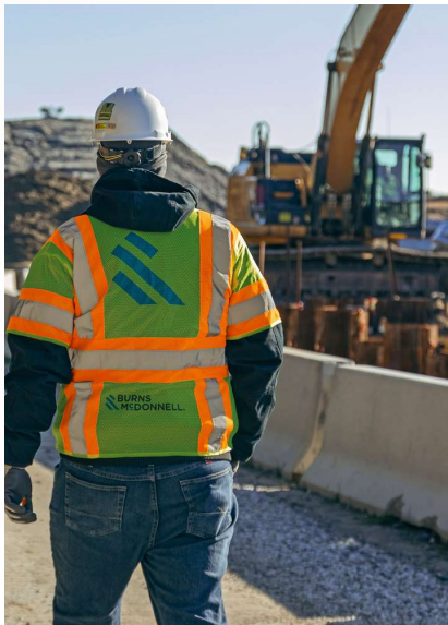
Example #1: Underground Service Work
