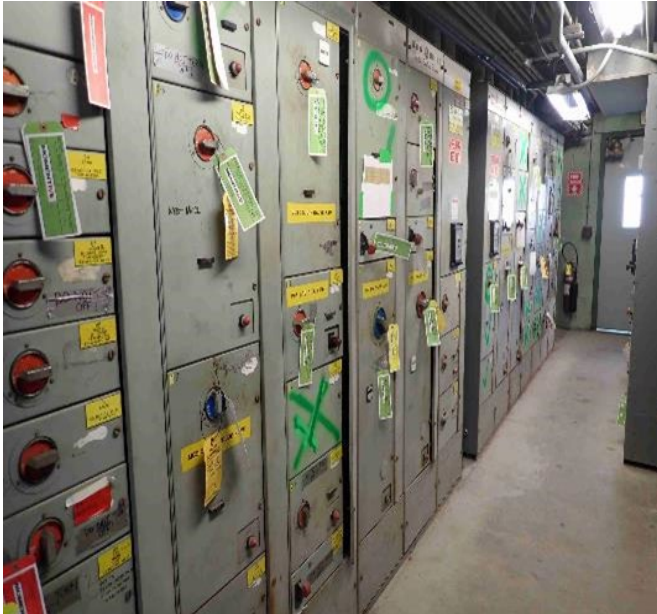
MCCs/breakers disconnected and de-energized
