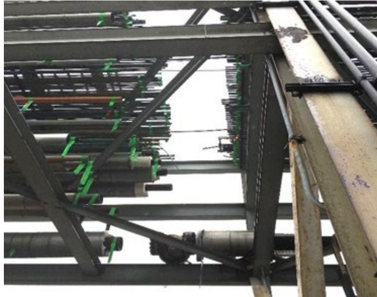
Utilities air gapped in pipe rack
