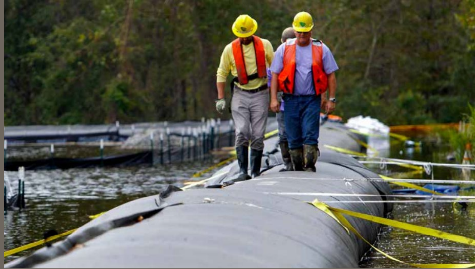
Grainger Ash Pond 2 – AquaDam installation
