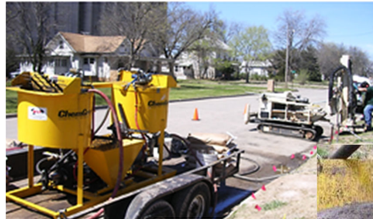
ZVI and amendments prepared as a slurry using a Grout Plant and injected directly through DPT drill rods
