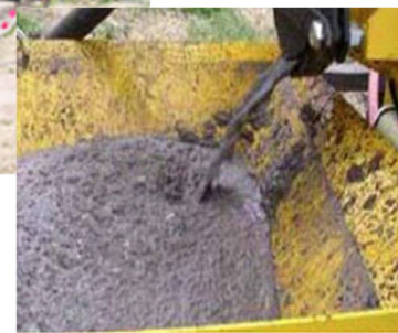
ZVI and amendments prepared as a slurry using a Grout Plant and injected directly through DPT drill rods
