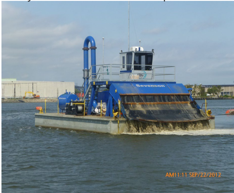
Hydraulic Placement of Cap Material
